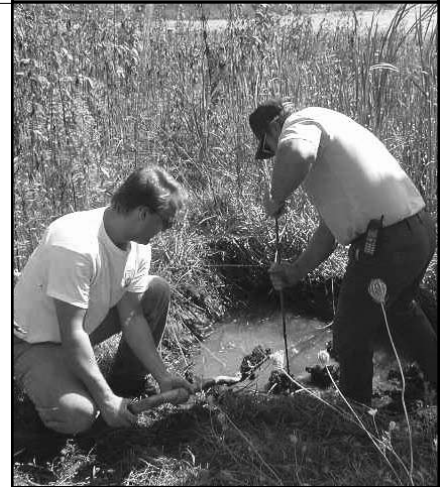
Learn about grants for wetland restoration techniques, like disabling drain tiles (above), at the seminar. Photo courtesy of Liberty Prairie Conservancy.
